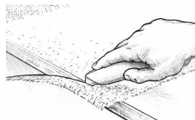
Figure 26 Trim excess cloth after the epoxy gels.
