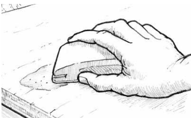
Figure 8 Sand non-porous surfaces. Provide a texture for epoxy to key into.
